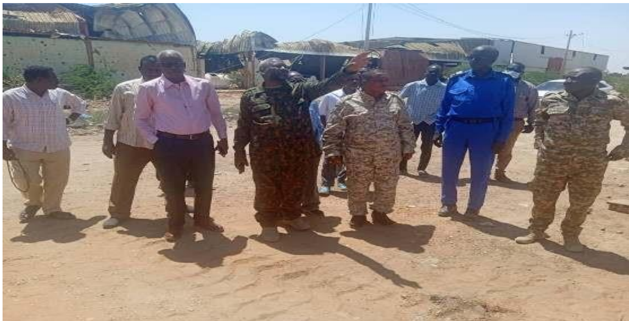
Top government officials and senior police officers oversee the demolition operations
