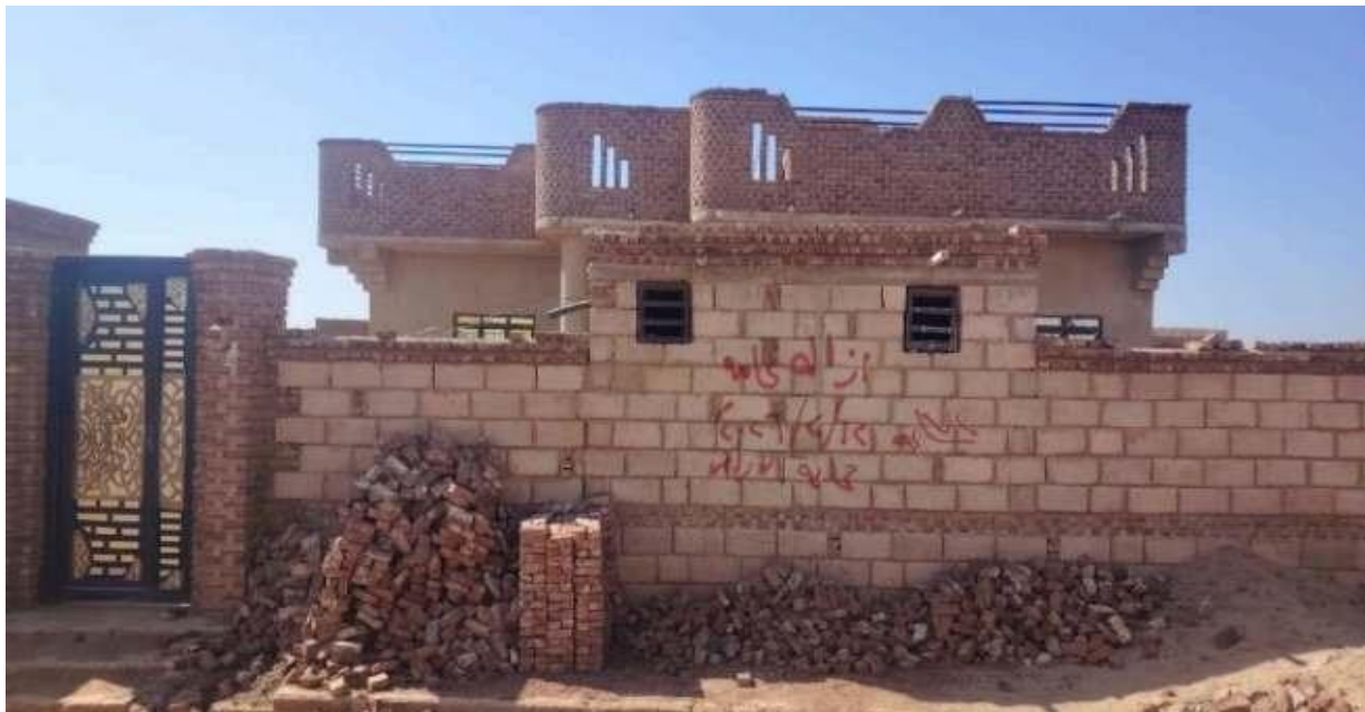
A house under construction earmarked for demolition in Khartoum North
